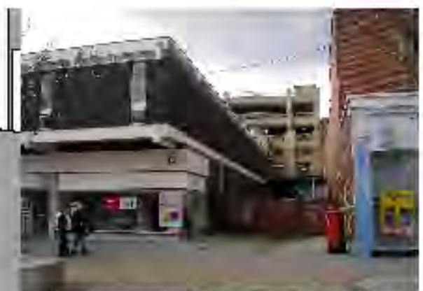
PHOTO 1 VIEW OF POTENTIAL ENTRANCE AREA TO CAR PARK FROM HIGH STREET
